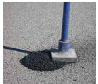
3. Compact PPR - job done!
