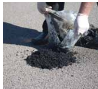
2. Apply PPR in to pothole
