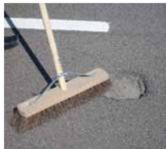
1. Ensure pothole is free of debris
