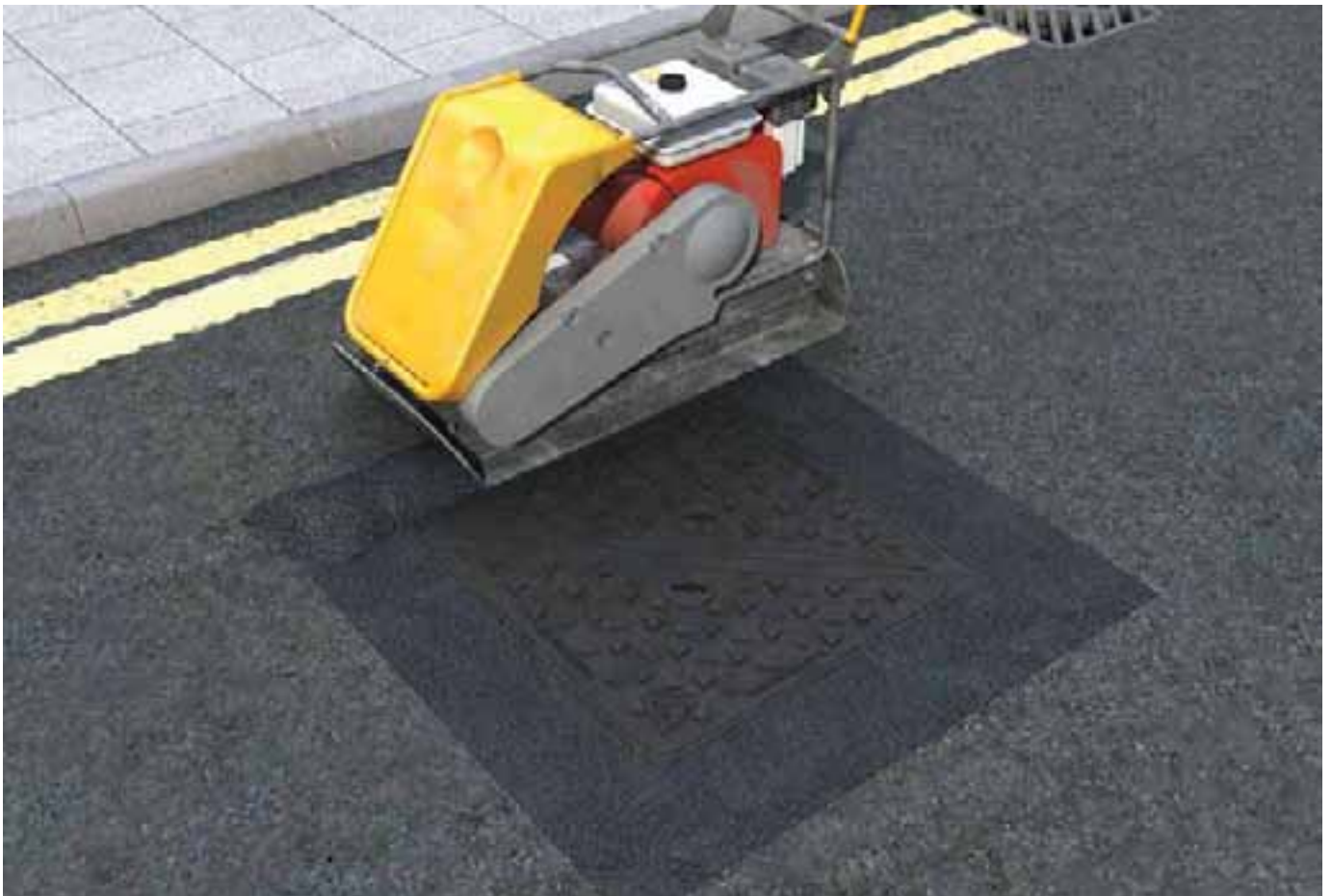
Reinstated Manhole
