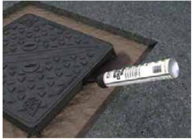
Stage 3 - Bitumen Sealer Spray
