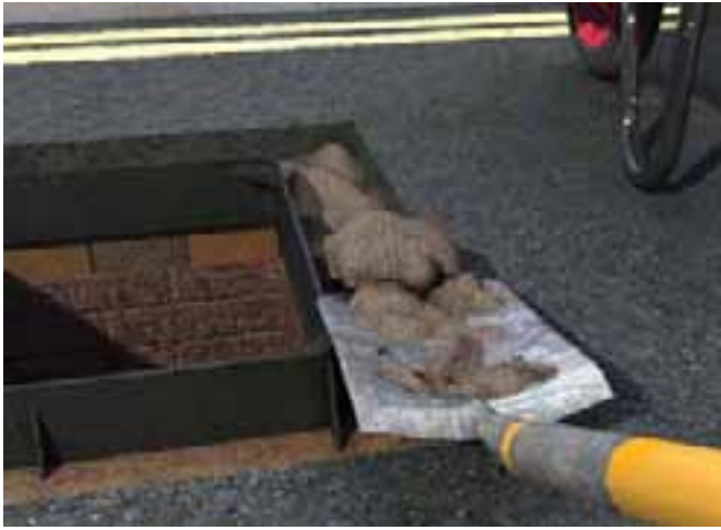
Stage 2 - Backfill Concrete
