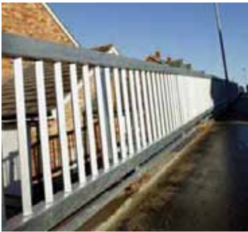
N1 Parapets Low Speed
