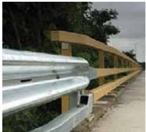
Transitions Connection to Safety Barriers
