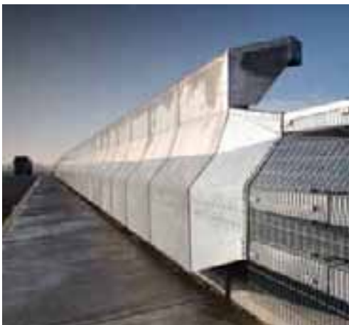
H4a Parapets Very High Containment
