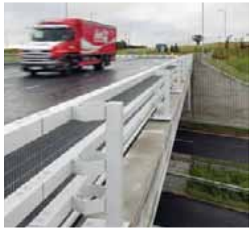
N2 Parapets Normal Containment
